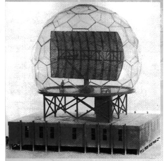
Model of the Sentinel radar, a long-range Doppler-capable automatic-alarm radar operating at 600 MHz, 3-kW average power, part of the DEW Line system, 1955.
