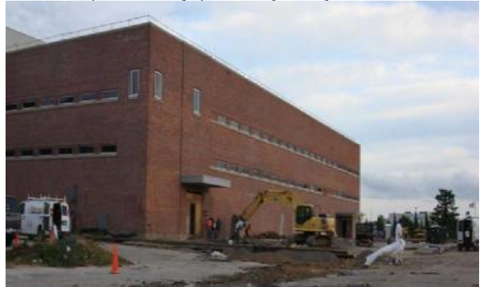
Construction Progress Continues at the Bethpage Facility
