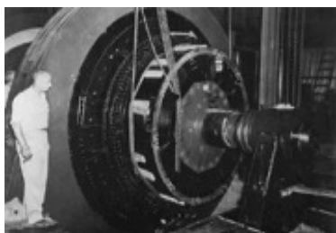
Panama Canal Electrical & Control Installations
