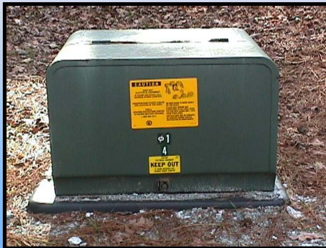
Single Phase Pad Mounted Transformer
