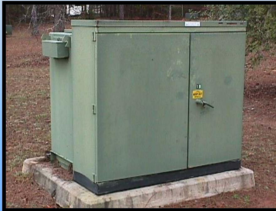
Three Phase Pad Mounted Transformer
