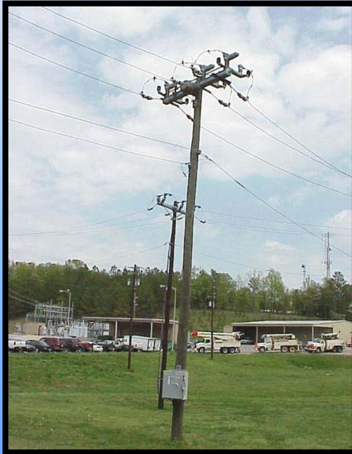
Gang Operated Switch with Motor Controls
