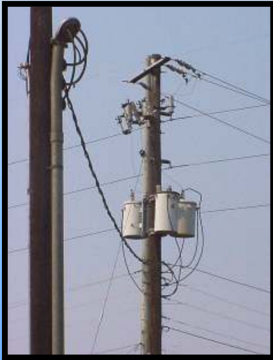
Overhead Transformer Bank & Service
