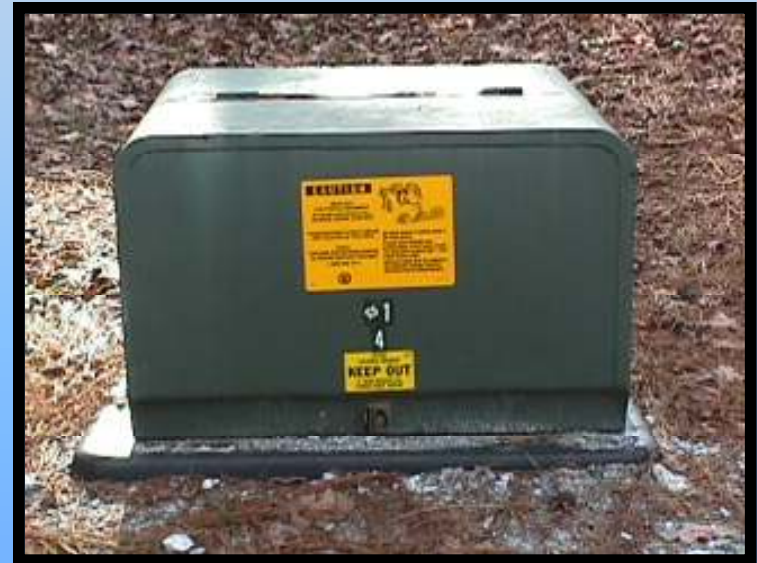
Padmount Transformer for Underground System
