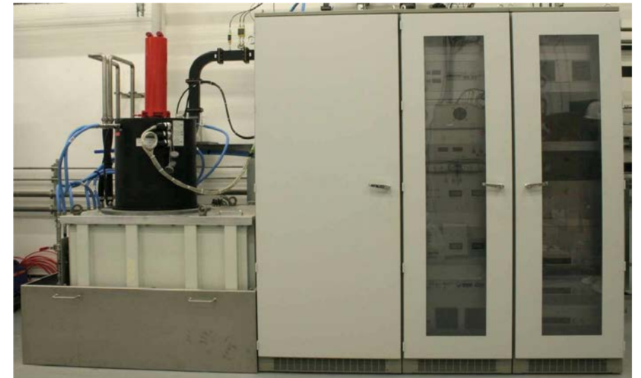
Solid-state klystron modulator National Synchrotron Light Source II
