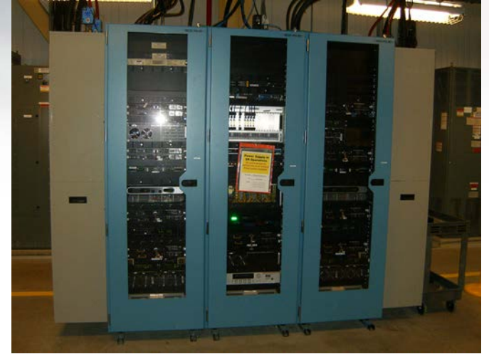
Multiple low-voltage power supplies
