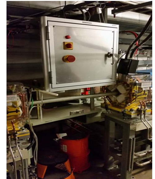
500 ns 20 kV pulse generator
