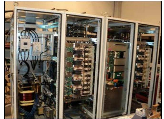
0.5 MW ramping power supply
