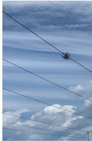
Kinectrics' robot on NY T-line
