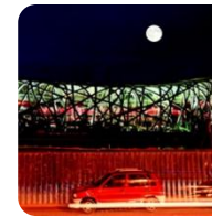
Structural Health Monitoring
